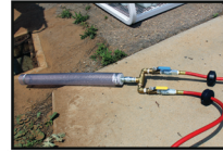
Lubrication Injection Manifold
